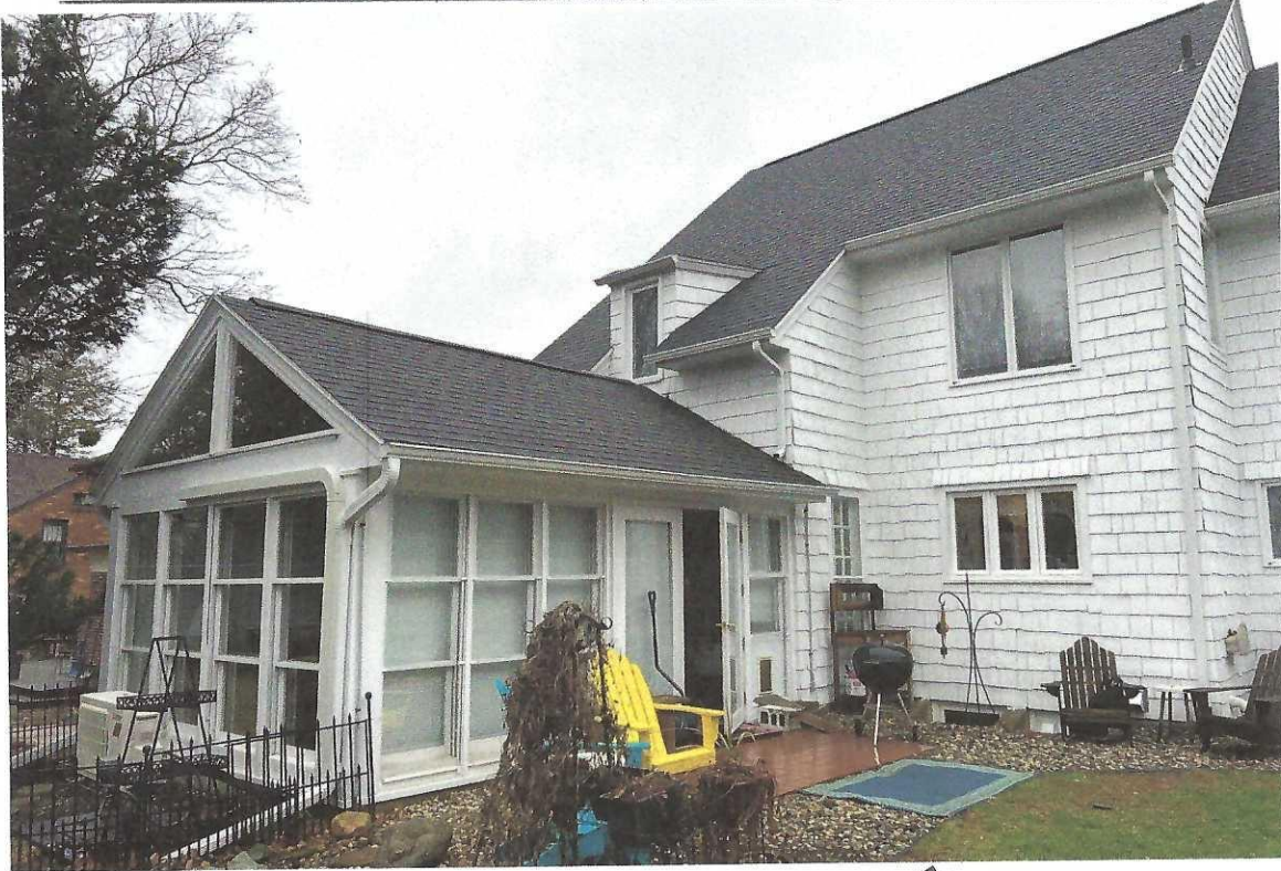
REAR YARD VIEW OF ADDITION ↗
