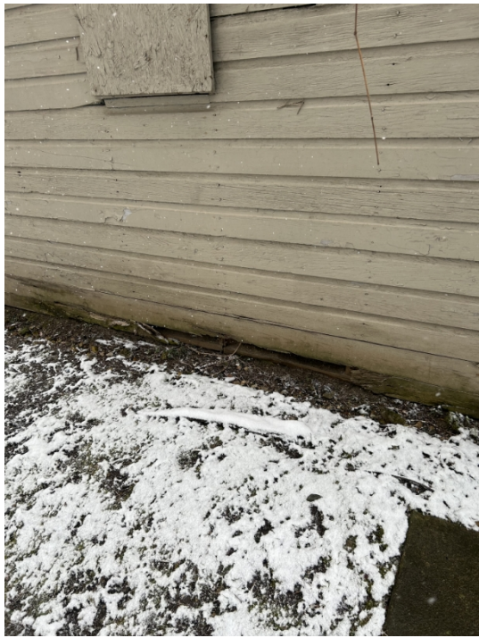
(1) 1105 S Park Garage – Looking SW (Detail)
