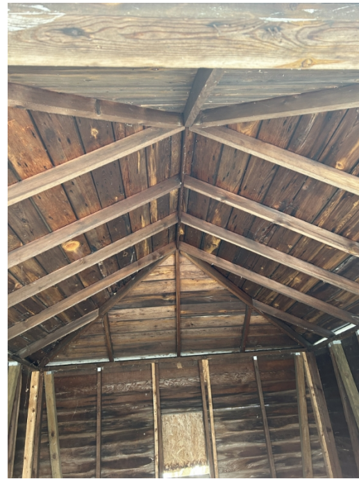
(2) 1105 S Park Garage ceiling
