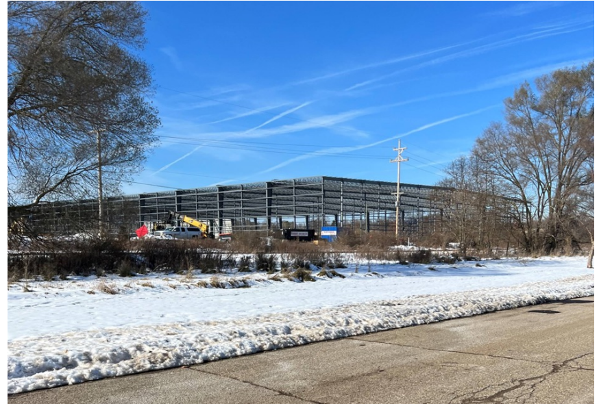
IP USA Speculative Building – Milham Road – Kalamazoo
