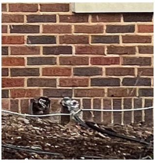
Existing Brick To be Reused
