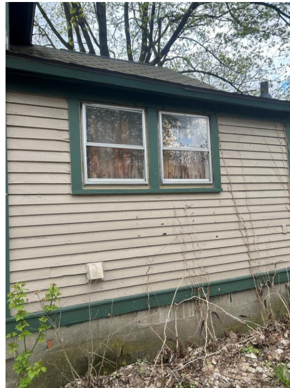
(2) 516 Oak Looking west, garage (4) 516 Oak looking south – first story windows
