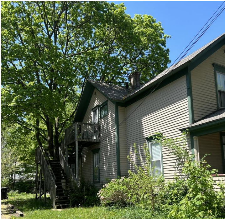
(1) 516 Oak– (above) Looking West (3) 516 Oak Looking north west – second story window
