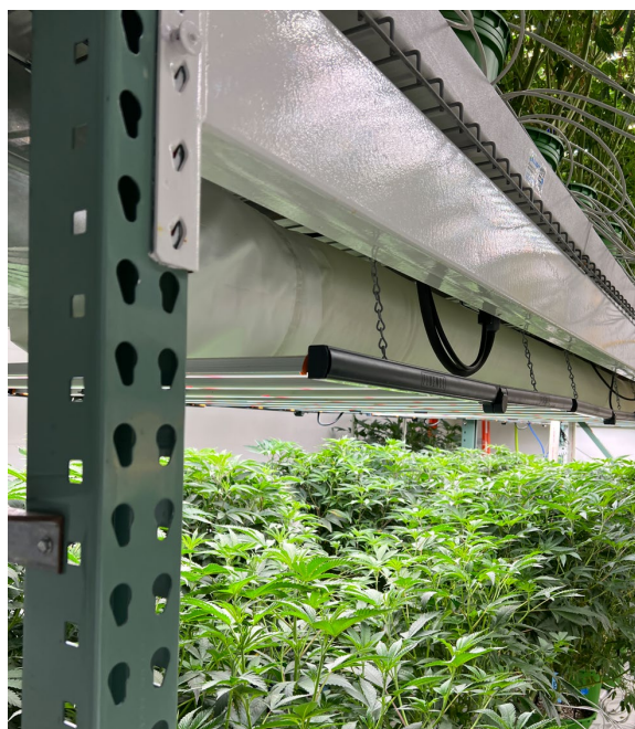
Figure 11. Vegetative Room SPYDR 2p47 LEDs running 15% wattage
