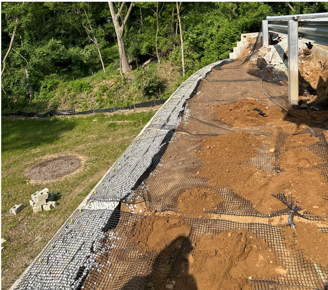
Photograph #2: The retaining wall while the repairs were in progress. (Gage Provisional Center Retaining Wall, Kalamazoo, Michigan, June, 2023)
