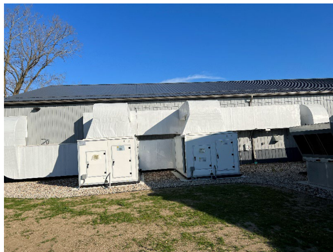
Figure 2. High efficiency units serving Flower Room 3 (2 units serve the room)
