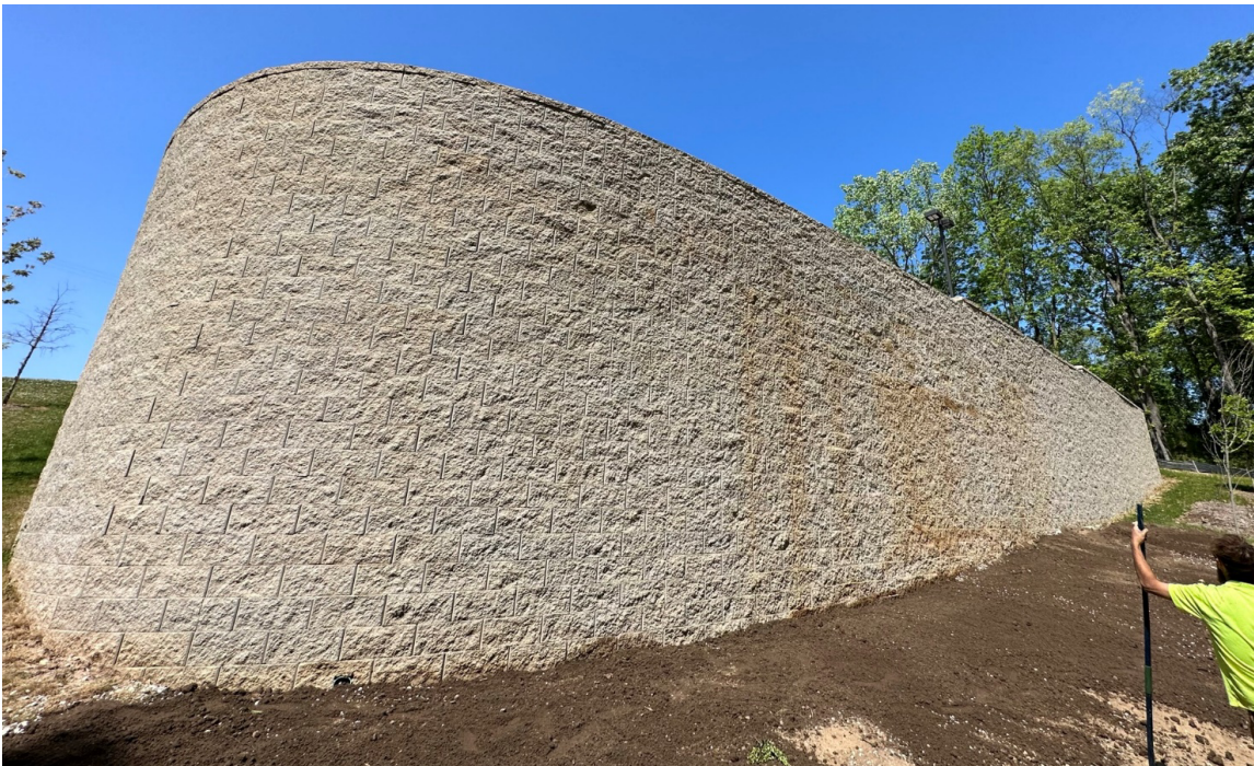
Photograph #1 The south face of the retaining wall after the repairs were completed. (Gage Provisional Center Retaining Wall, Kalamazoo, Michigan, June, 2023)
