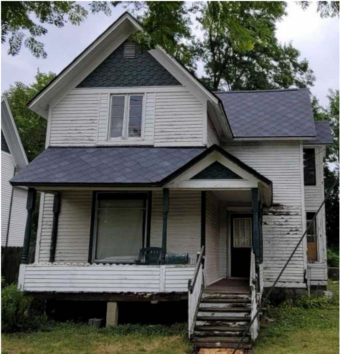
Picture 1: 712 Willard, June 2021 showing porch configuration
