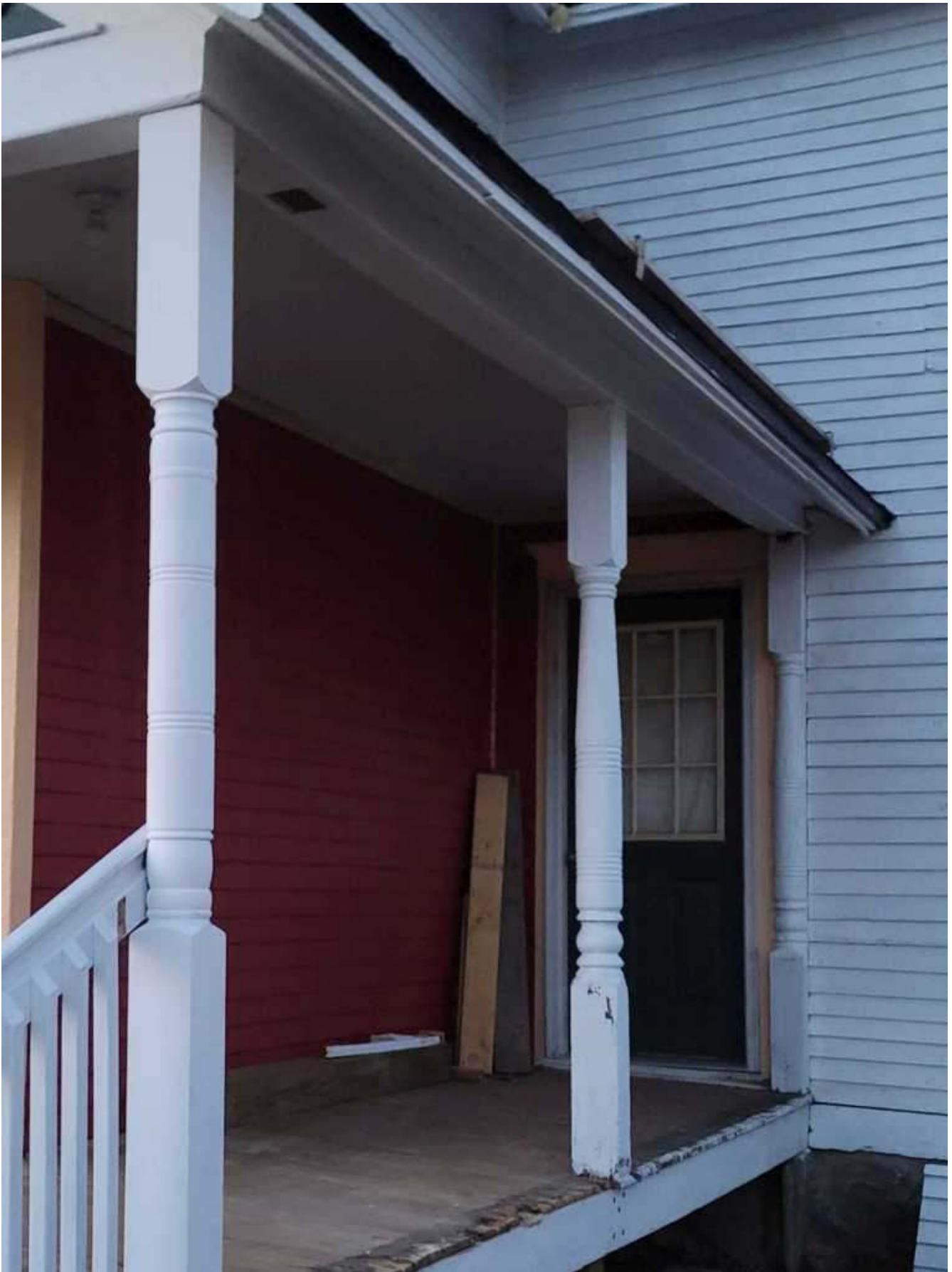
Picture 4: Turning detail on new vs original column
