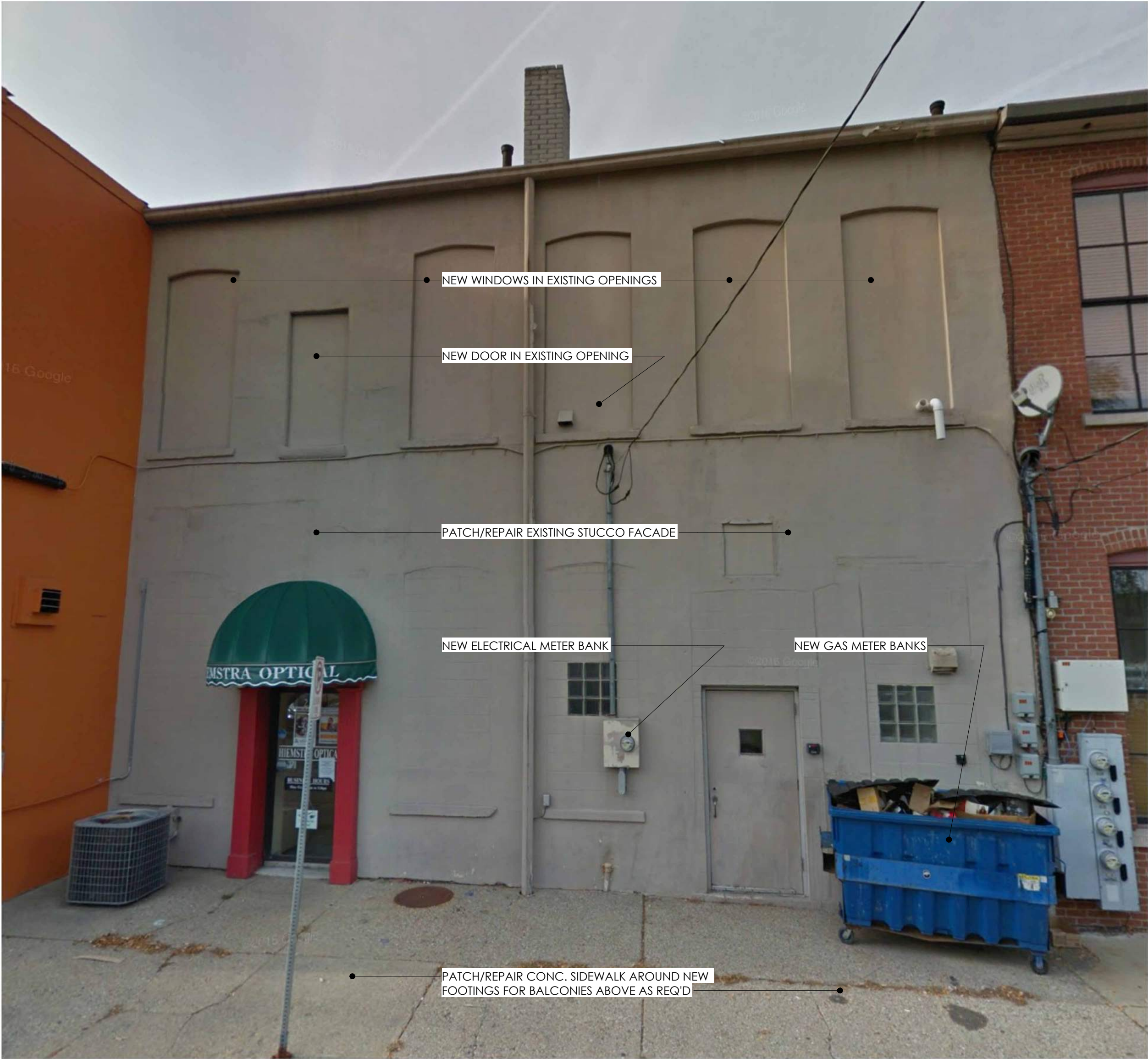
EXISTING REAR FACADE - FOR REFERENCE ONLY
