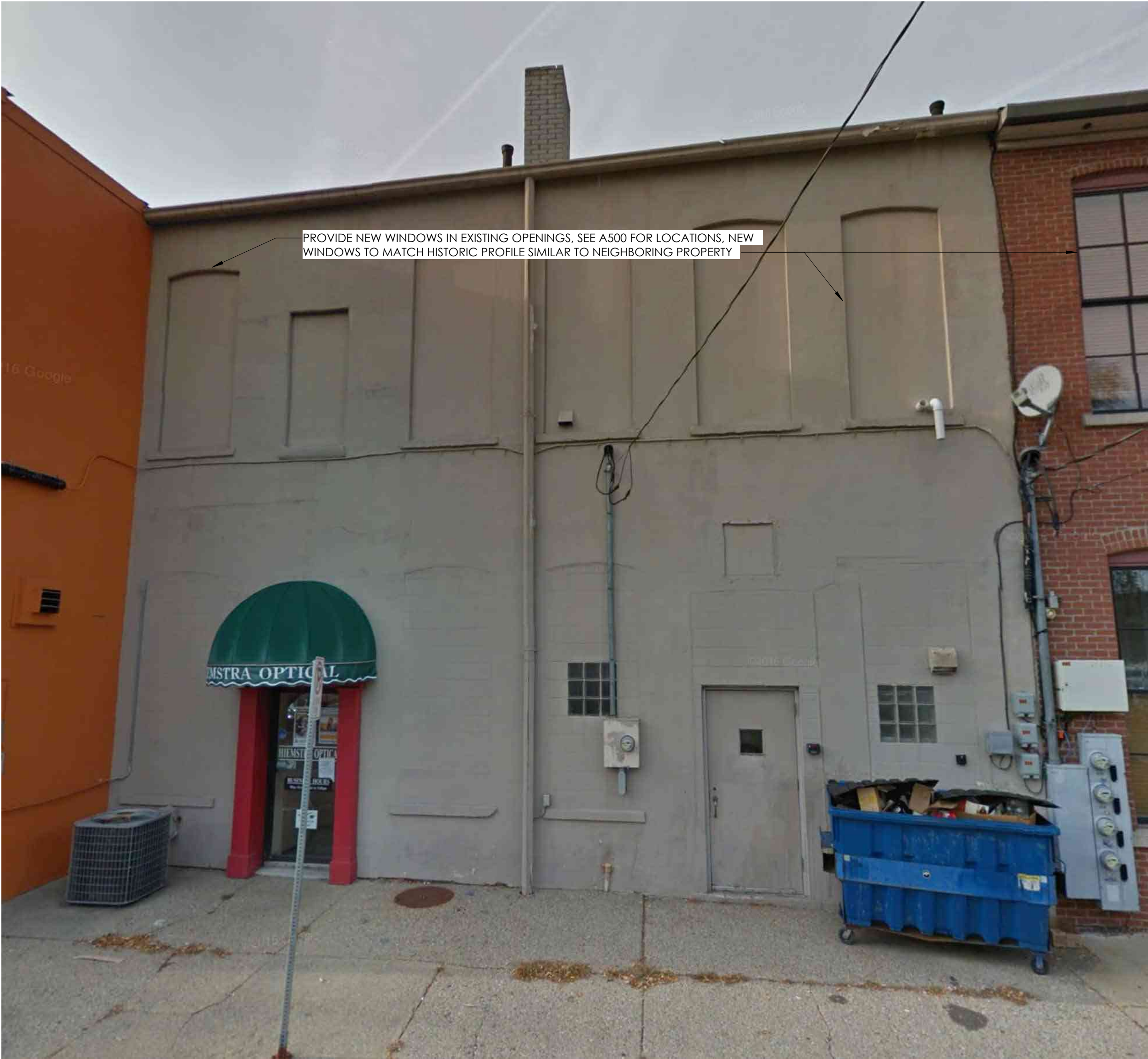
EXISTING REAR FACADE - FOR REFERENCE ONLY
