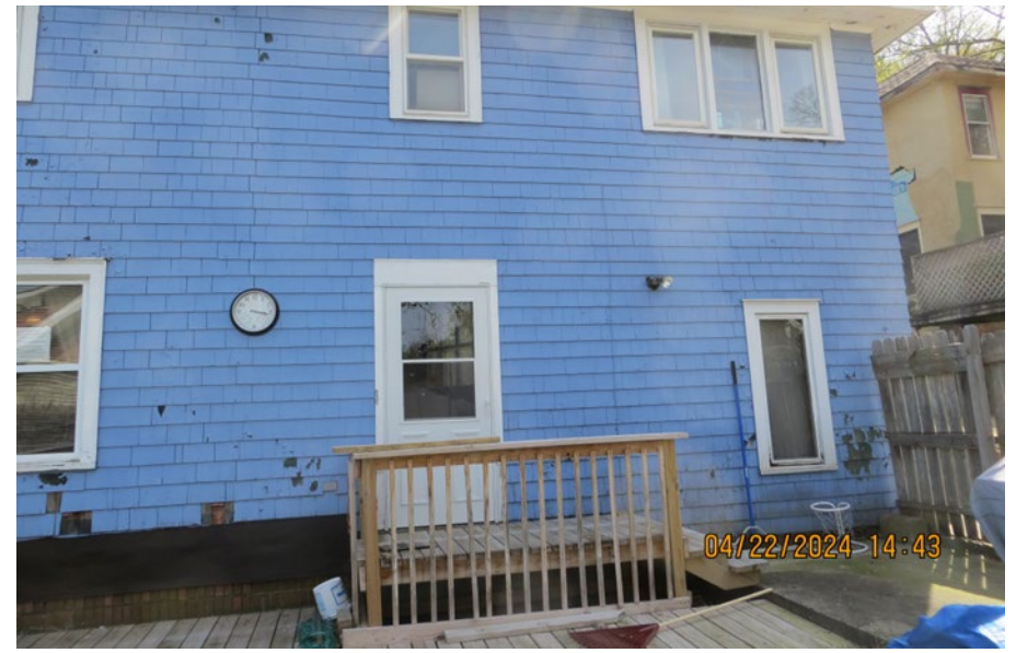
North side – NW corner.- single lite 1 st floor window to be removed
