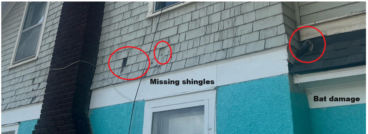
Shake siding replacement (original part of house) - Menards Allura 0.25" x 16" x 48" fiber cement straight edge shake siding ($10.89 each)
