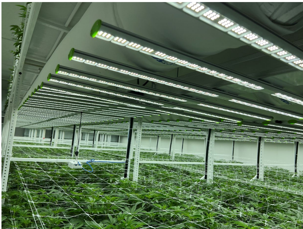
Figure 11. Vegetative Room SPYDR 2p47 LEDs running 15% wattage
