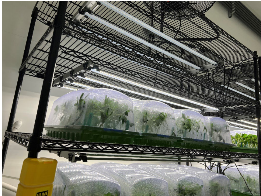
Figure 12. Fluence RAZR LEDs in Clone Room
