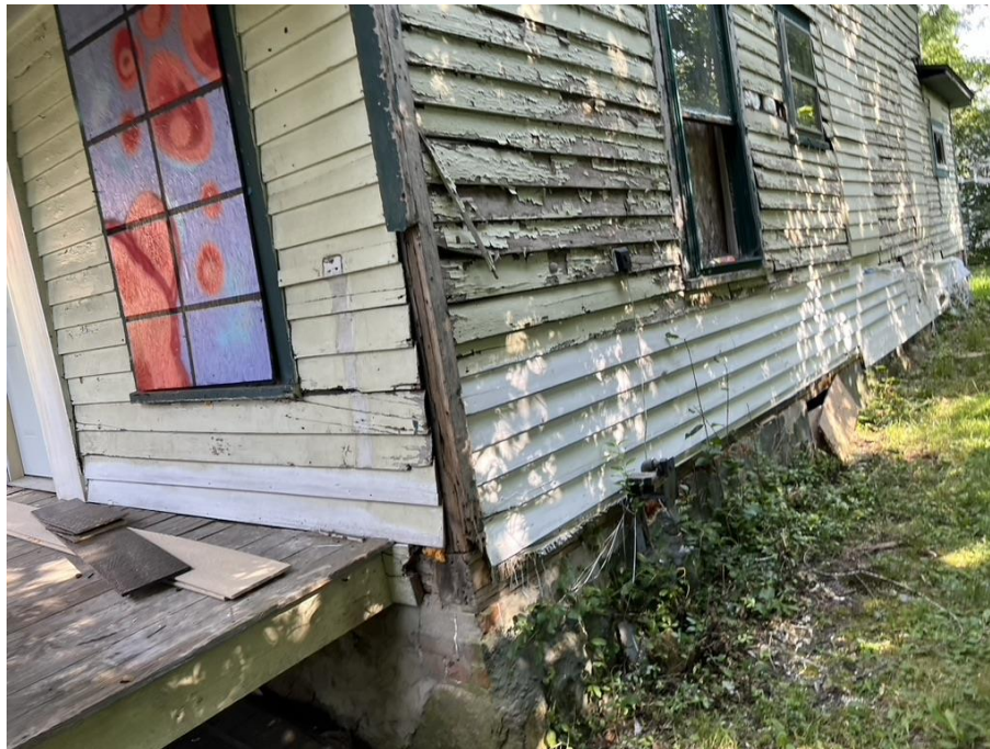
West Side View (1)
