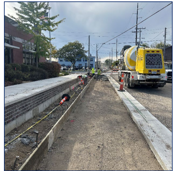
Figure 1: Concrete for bump-out and parking areas being poured near Metro.
