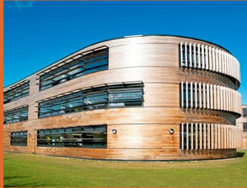
Langley Academy, Berkshire Foster + Partners
