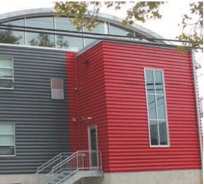
METAL SIDING - HORIZONTAL
