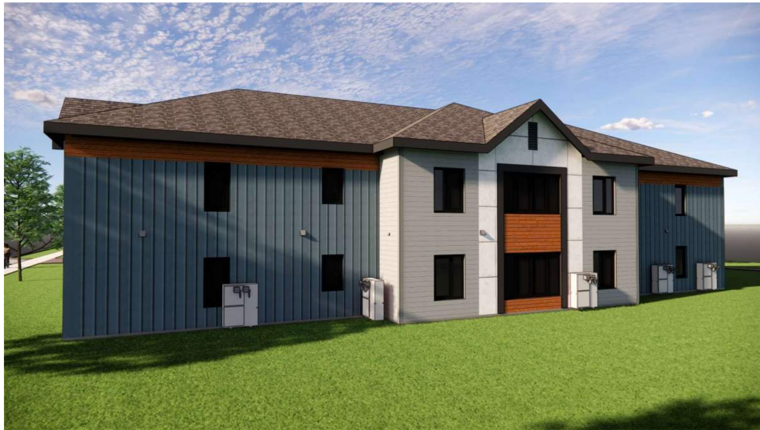
NORTH PERSPECTIVE : BUILDING B ( BLDG. C SIMILAR)
