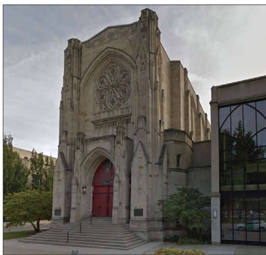
First Presbyterian Church Source: Google Street View
