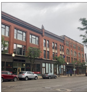
A row of historic mixed-use Haymarket District buildings
