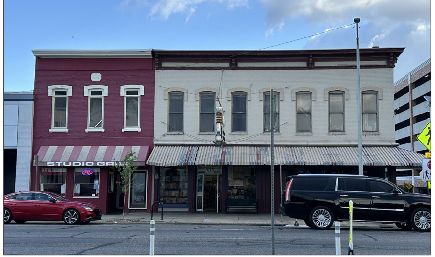
Fabric buildings on W. Michigan Avenue at Church Street
