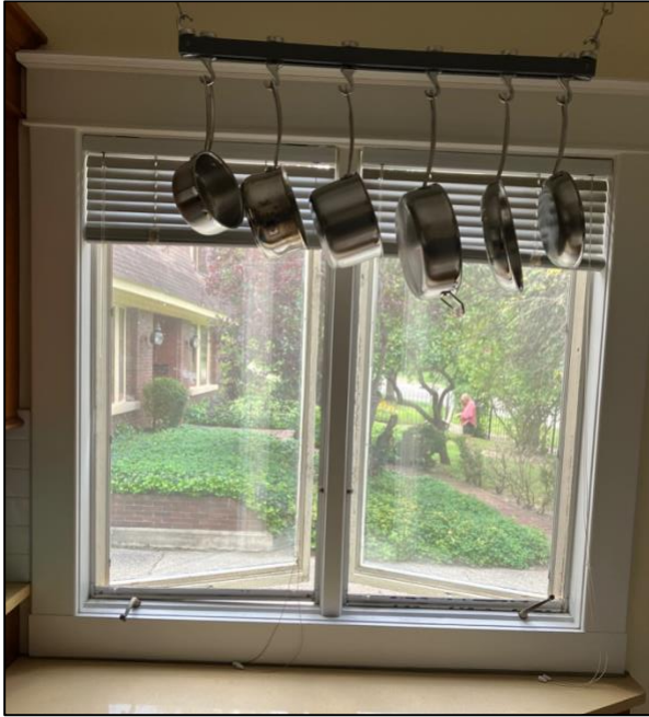
Interior view of the window
