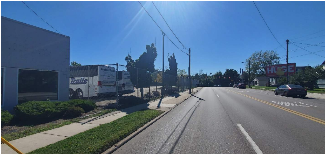
Existing 10' Security Fencing along Riverview Dr.
