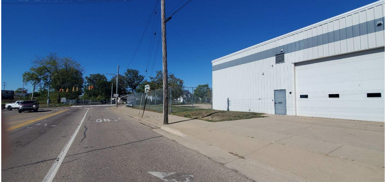
Existing 10' Security Fencing along Michigan Ave.
