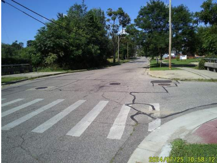
Document Name: DSCF0011.JPG Category: Approach Span Number: Comments: Looking west
