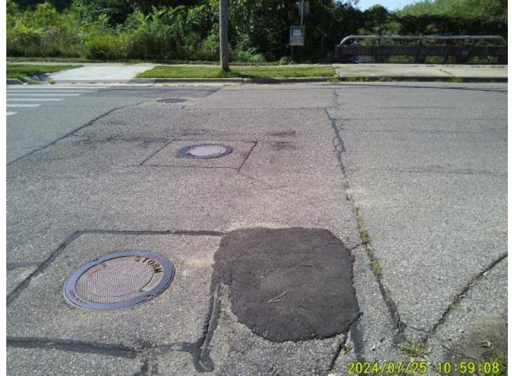
Document Name: DSCF0012.JPG Category: Approach Span Number: Comments: East approach, looking south
