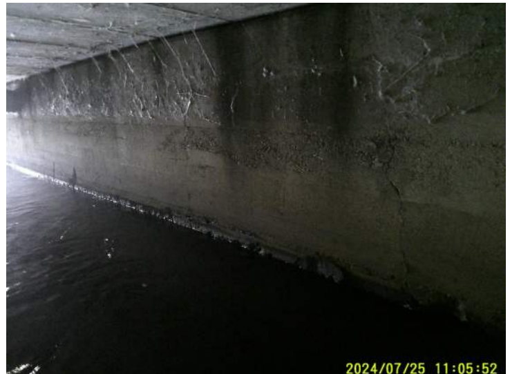
Document Name: DSCF0013.JPG Category: Substructure Span Number: Comments: West abutment, crack near centerline
