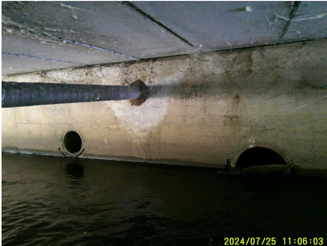
Utility Line and storm sewer outlets
