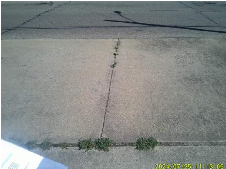
Document Name: DSCF0016.JPG Category: Deck Span Number: Comments: South sidewalk
