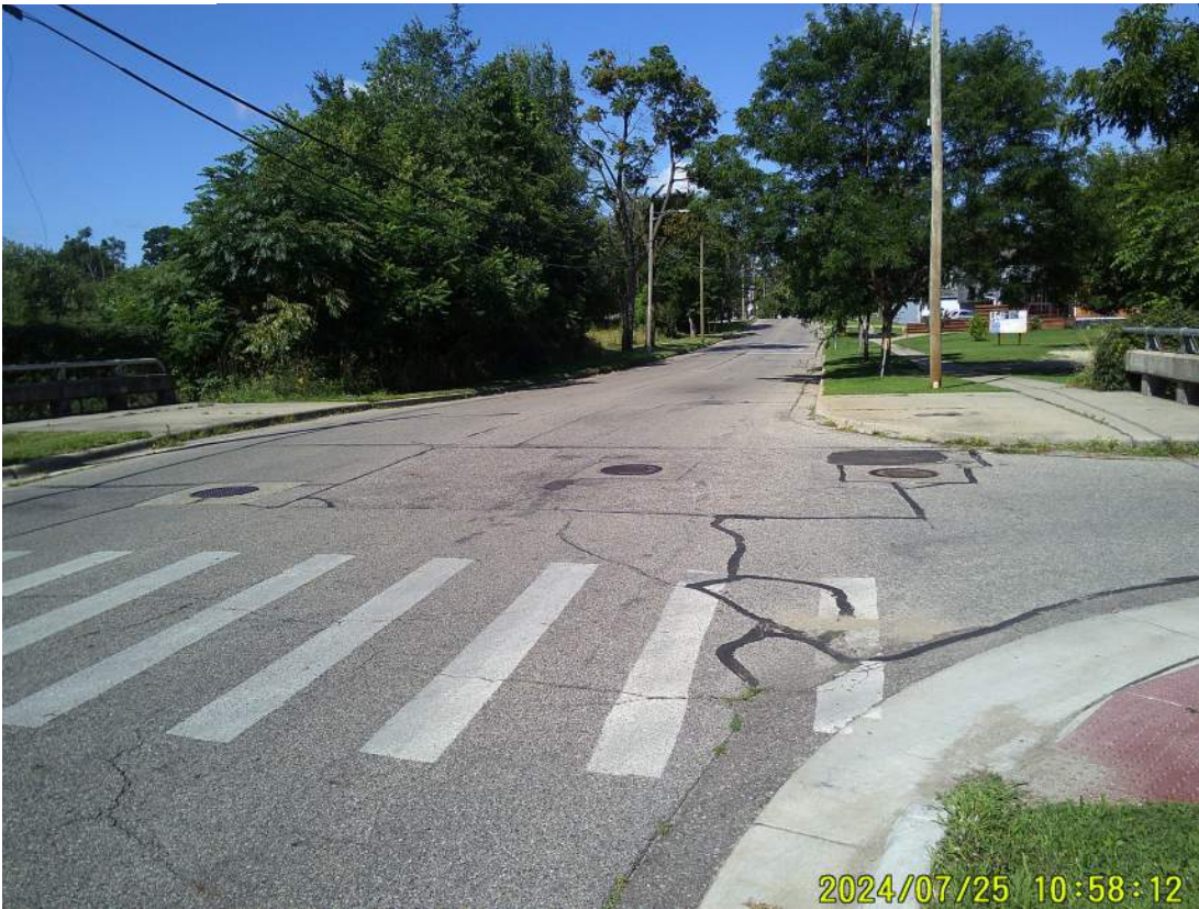
Approach Looking West
