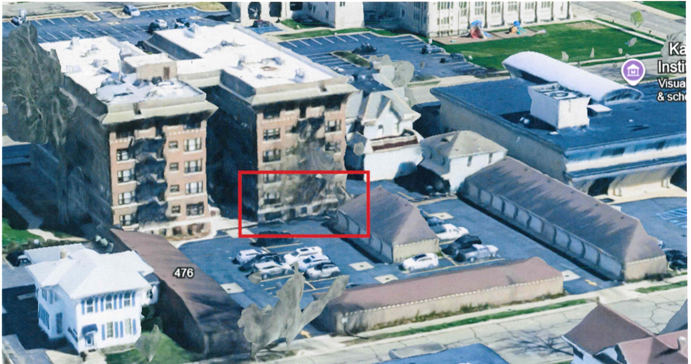
AREA OF WORK – SOUTH ELEVATION / EASTERN LEG
