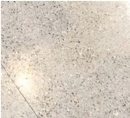
GROUND CONCRETE FLOOR
