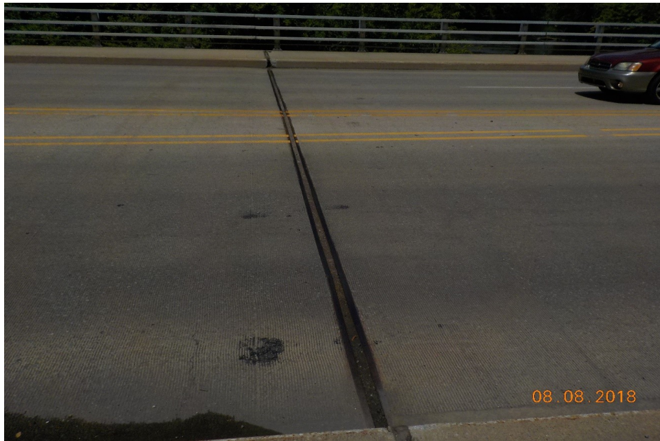
Pier 1W joint
