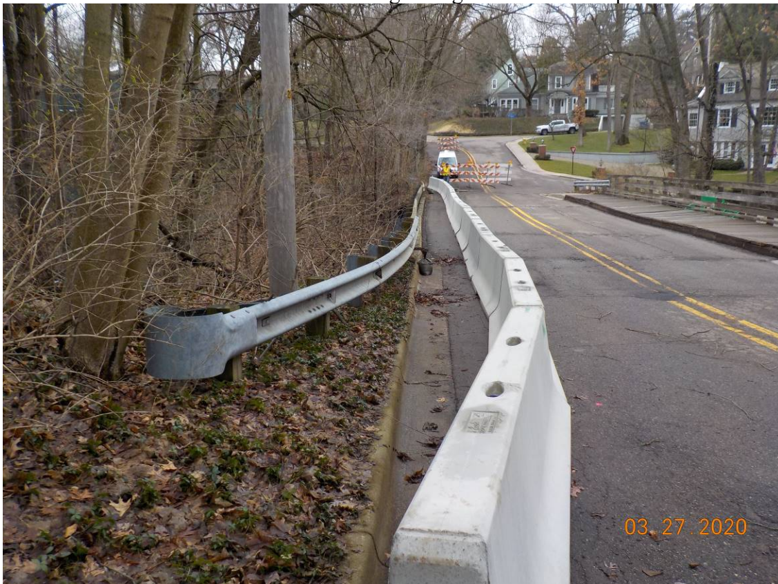
Barrier to protect south railing
