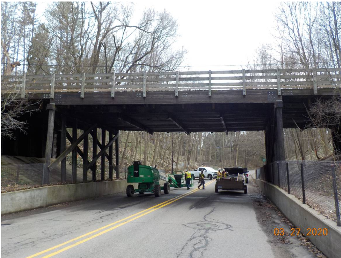
North Elevation after bearing re-alignment and end repairs
