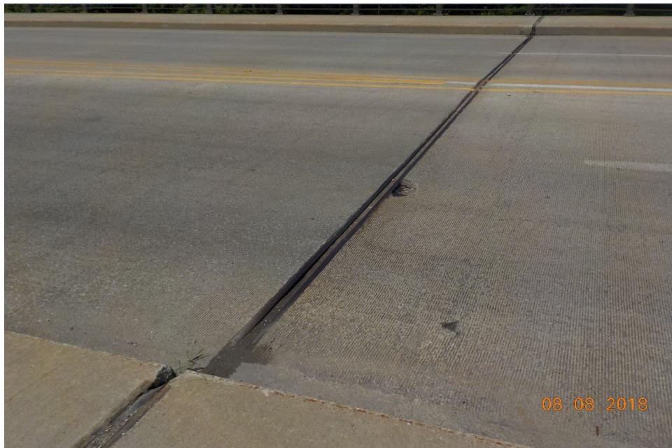
Pier 2W joint
