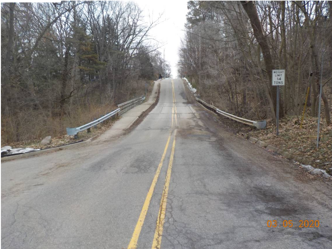
East approach looking west
