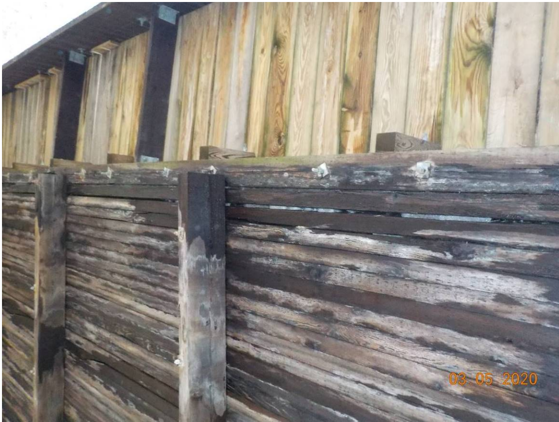
Under center span, north sidewalk, looking east
