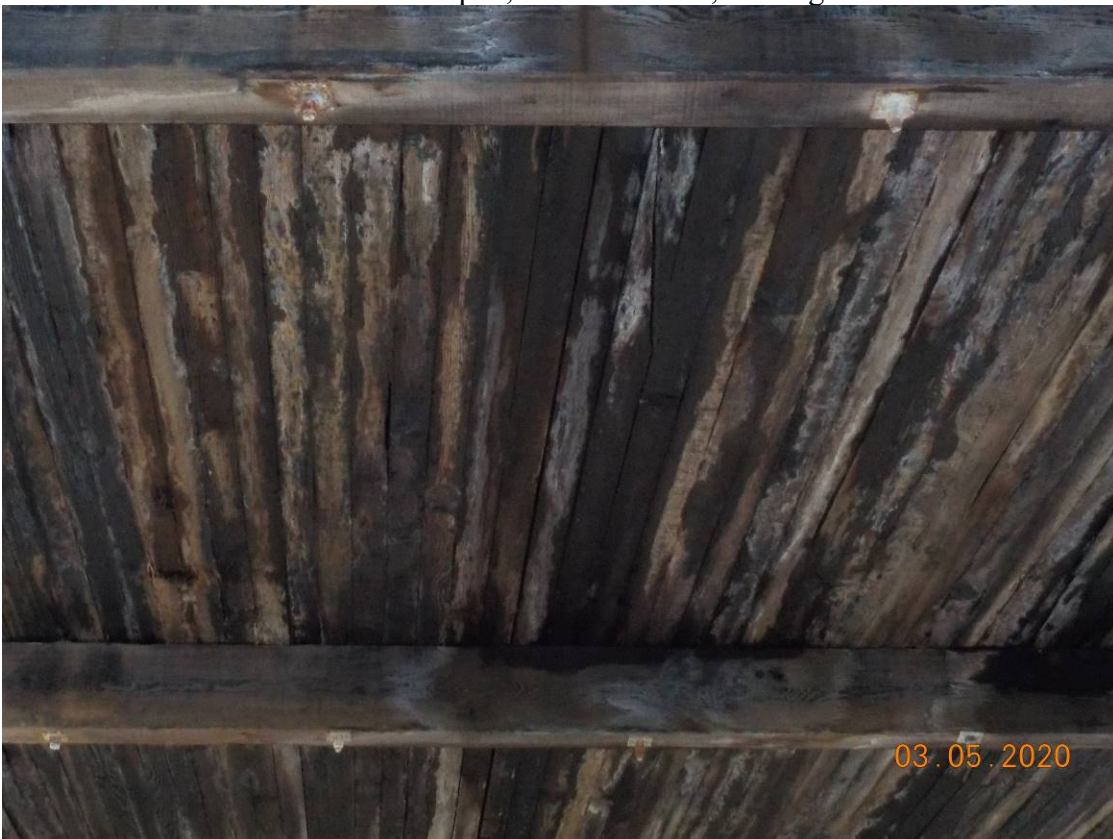
Timber panels center span, Panel 3S
