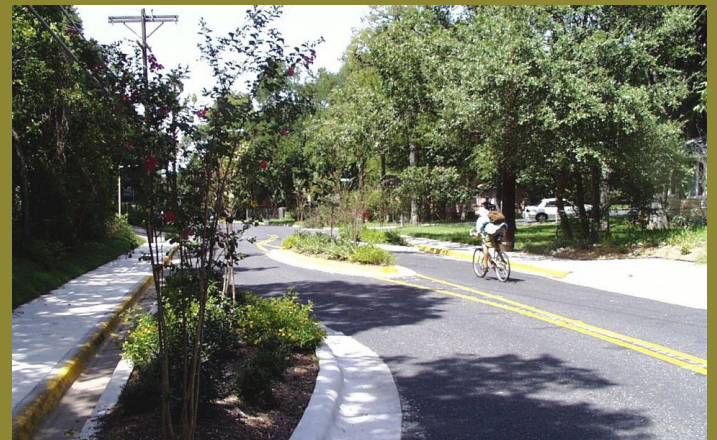
Chicane, Source: nacto.org/publication/urban-street-design-guide/street-design-elements/curb-extensions/chicane/
