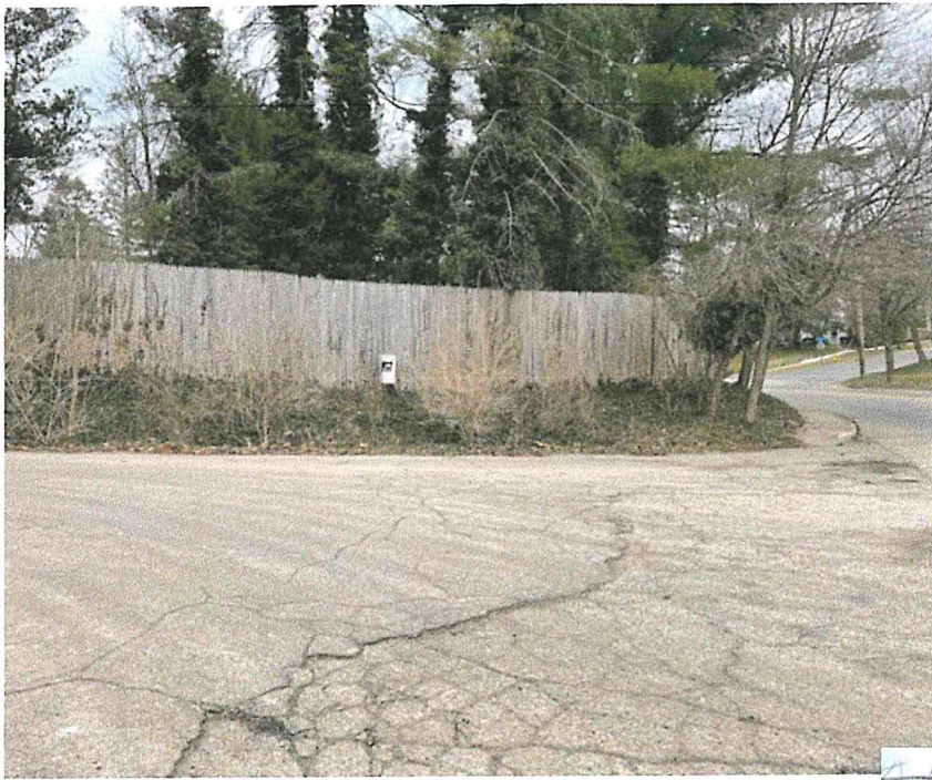
Alley #1 Fence runs perpendicular to Bronson. These panels are currently 8 ft.
